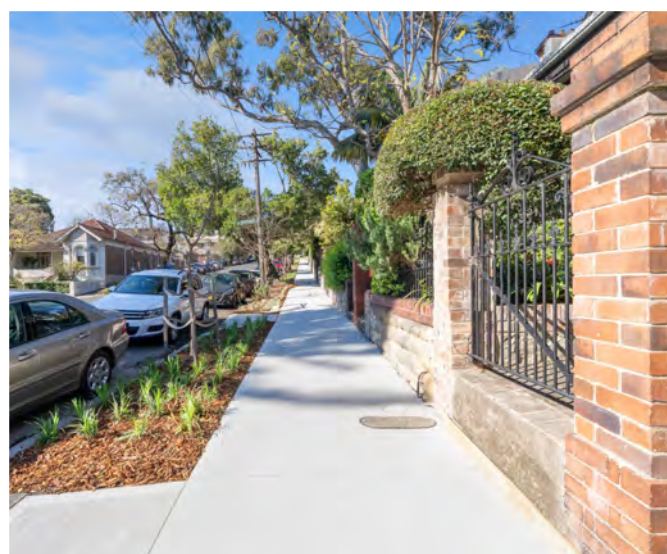
Images: Eglinton Road, Glebe Footpath Renewal Works 2021
